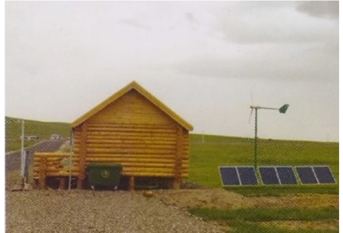
Fig. 13: Basic configuration of high-power wind-solar complementary power generation system
